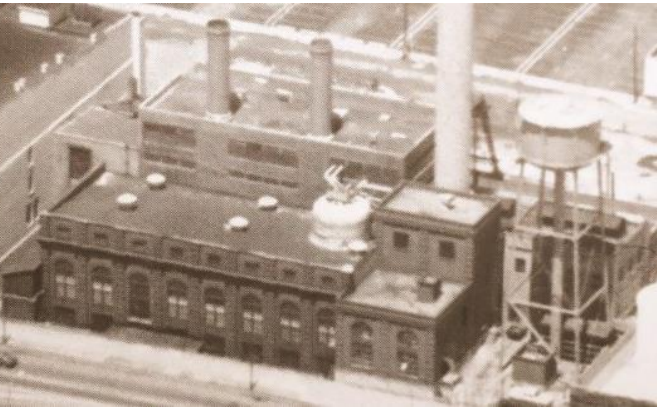
Built in downtown Dayton in 1907, this power-generating plant closed its doors in the mid-1980s.
