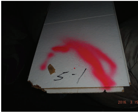
Sample 5-1 Ceiling Tile
