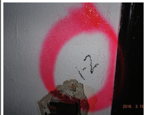
Sample 1-2 Plaster/Skim Coat
