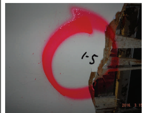
Sample 1-5 Plaster/Skim Coat
