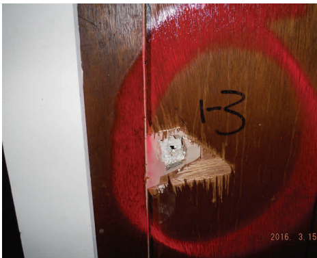
Sample 1-3 Plaster/Skim Coat
