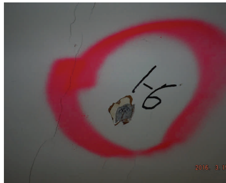
Sample 1-6 Plaster/Skim Coat
