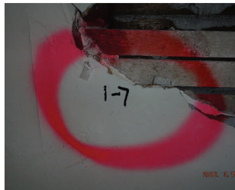
Sample 1-7 Plaster/Skim Coat
