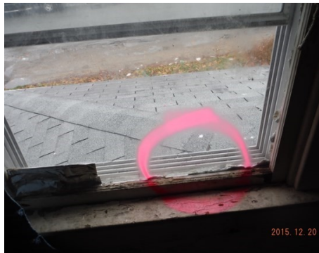
Sample 4-1 Window Glazing
