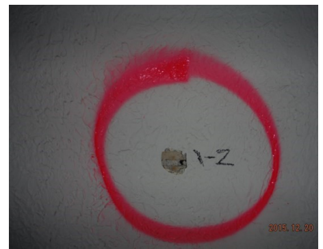
Sample 1-2 Plaster/Skim Coat
