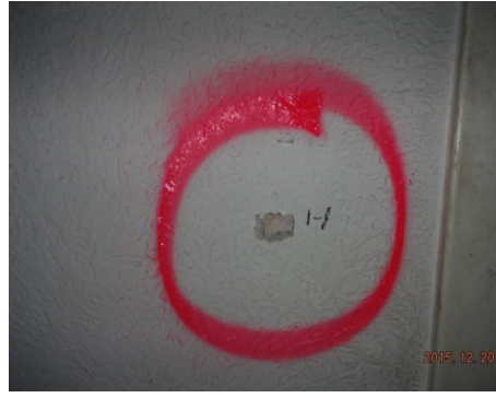
Sample 1-1 Plaster/Skim Coat
