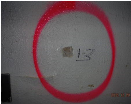
Sample 1-3 Plaster/Skim Coat
