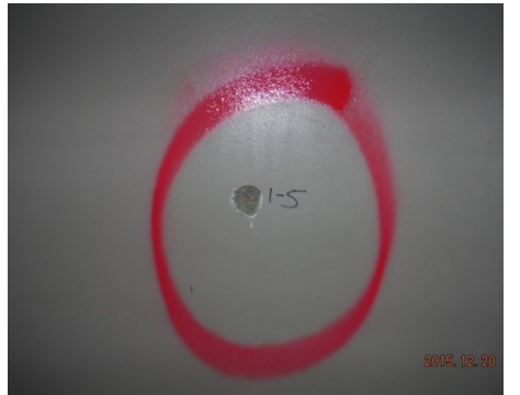
Sample 1-5 Plaster/Skim Coat
