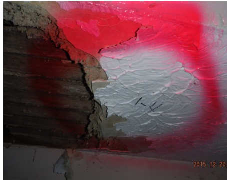
Sample 1-4 Plaster/Skim Coat
