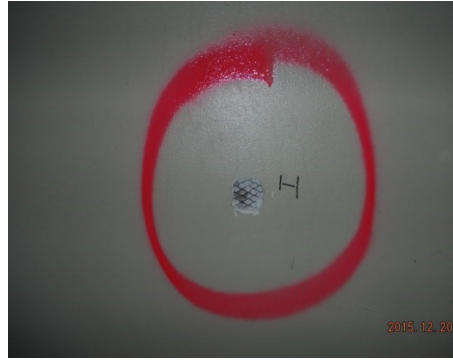
Sample 1-1 Plaster/Skim Coat
