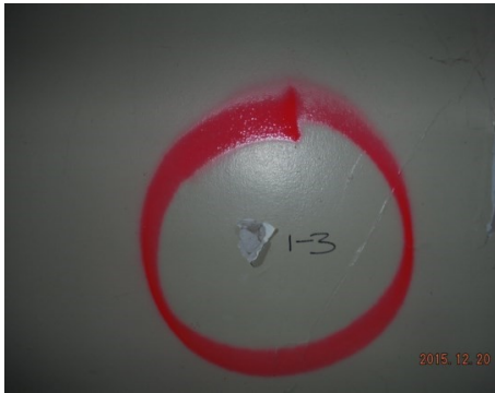
Sample 1-3 Plaster/Skim Coat
