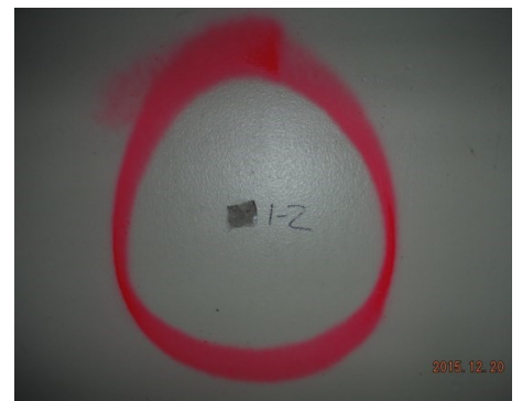
Sample 1-2 Plaster/Skim Coat
