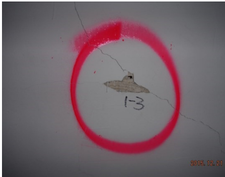
Sample 1-3 Plaster/Skim Coat
