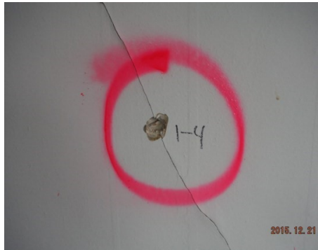
Sample 1-4 Plaster/Skim Coat
