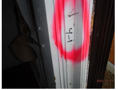
Sample 4-1 Window Glazing
