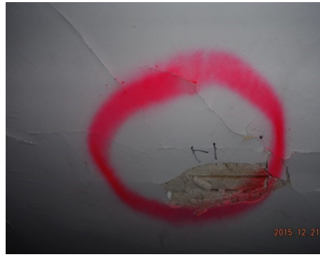
Sample 1-1 Plaster/Skim Coat
