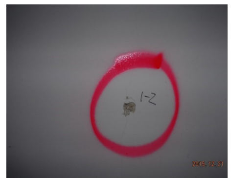
Sample 1-2 Plaster/Skim Coat
