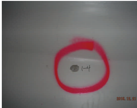
Sample 1-4 Plaster/Skim Coat
