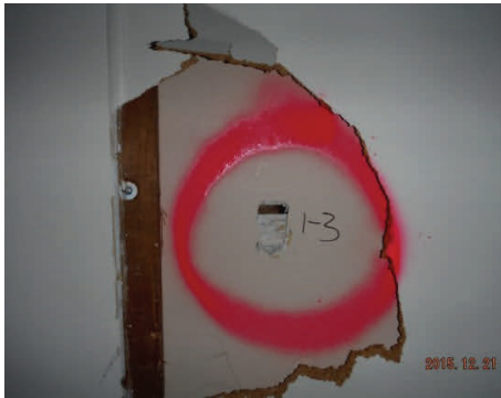
Sample 1-3 Plaster/Skim Coat
