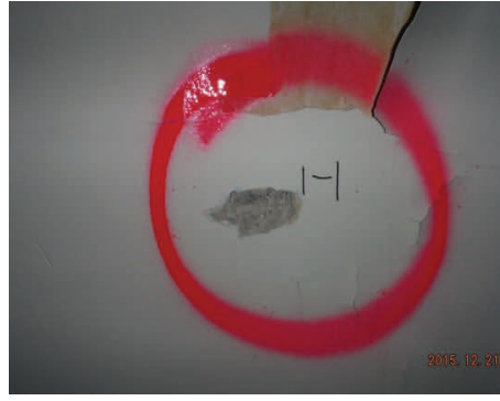
Sample 1-1 Plaster/Skim Coat
