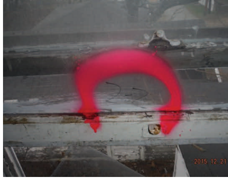
Sample 2-2 Window Glazing
