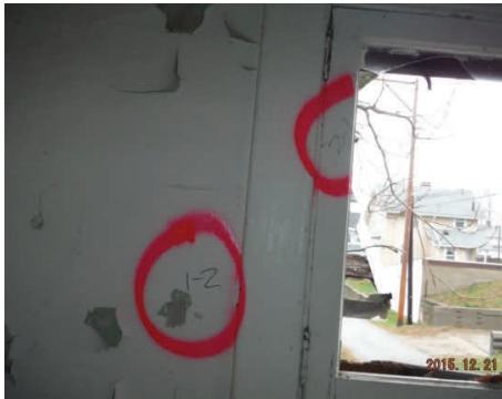
Sample 2-1 Window Glazing
