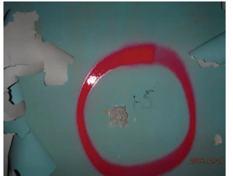
Sample 1-5 Plaster/Skim Coat
