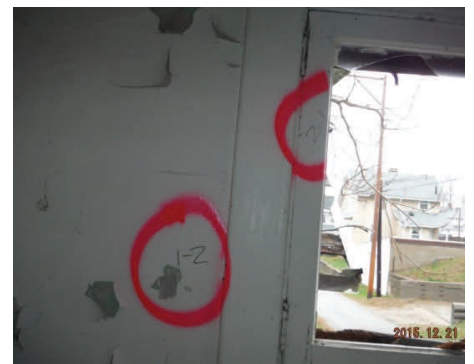
Sample 1-2 Plaster/Skim Coat
