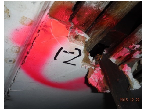
Sample 1-2 Plaster/Skim Coat
