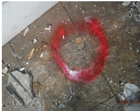
Sample 3-1 Floor Tile
