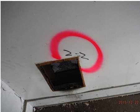
Sample 2-2 Duct Wrap
