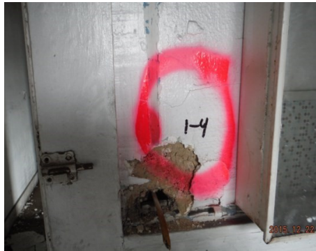
Sample 1-4 Plaster/Skim Coat
