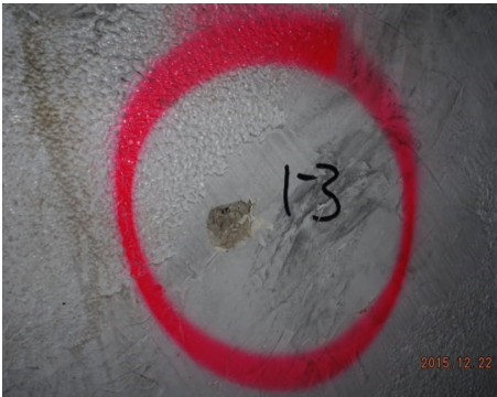
Sample 1-3 Plaster/Skim Coat
