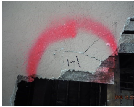
Sample 1-1 Plaster/Skim Coat
