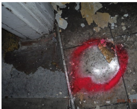
Sample 6-1 Floor Tile
