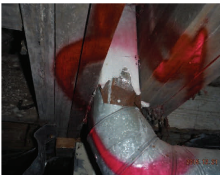
Sample 5-2 Duct Wrap
