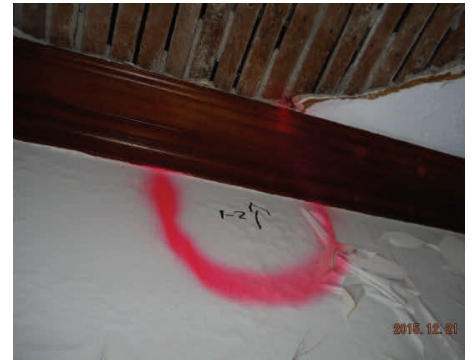
Sample 1-2 Plaster/Skim Coat
