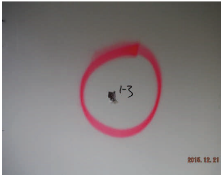
Sample 1-3 Plaster/Skim Coat
