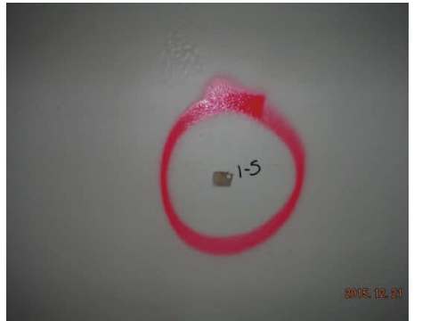
Sample 1-5 Plaster/Skim Coat
