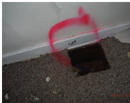
Sample 5-1 Duct Wrap
