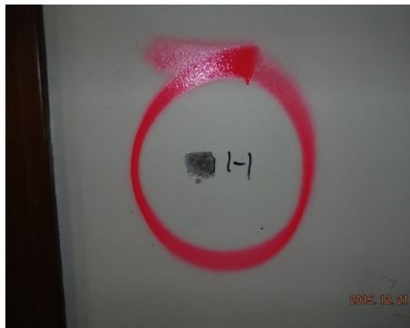
Sample 1-1 Plaster/Skim Coat
