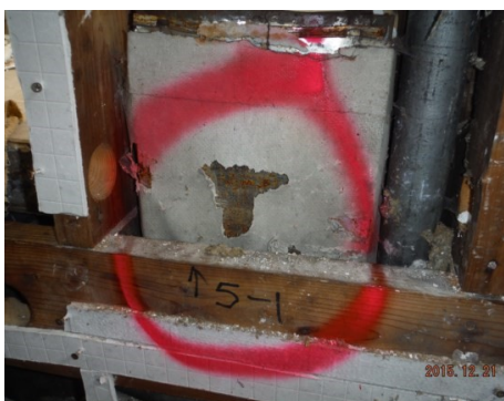
Sample 5-1 Duct Wrap
