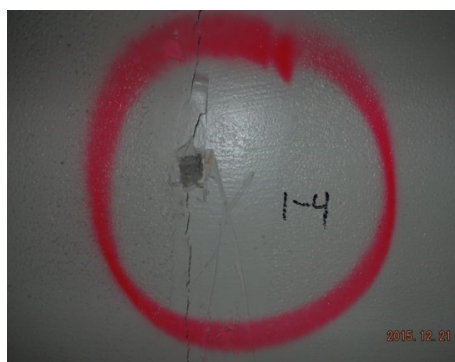
Sample 1-4 Plaster/Skim Coat
