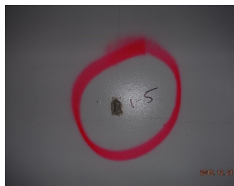
Sample 1-5 Plaster/Skim Coat
