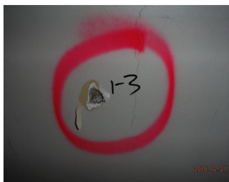
Sample 1-3 Plaster/Skim Coat
