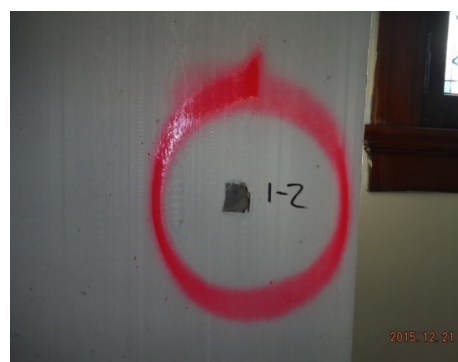
Sample 1-2 Plaster/Skim Coat
