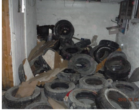
Clutter around basement Steps
