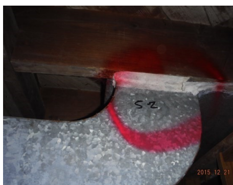
Sample 5-2 Duct Wrap
