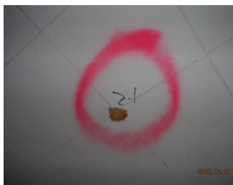
Sample 2-1 Ceiling Tile
