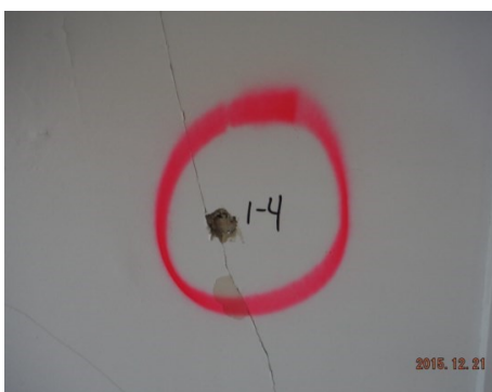
Sample 1-4 Plaster/Skim Coat
