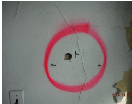
Sample 1-1 Plaster/Skim Coat
