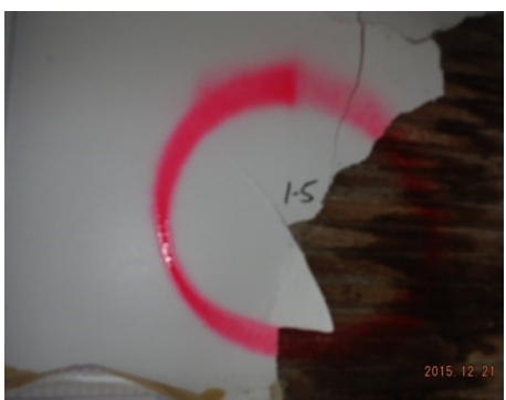
Sample 1-5 Plaster/Skim Coat
