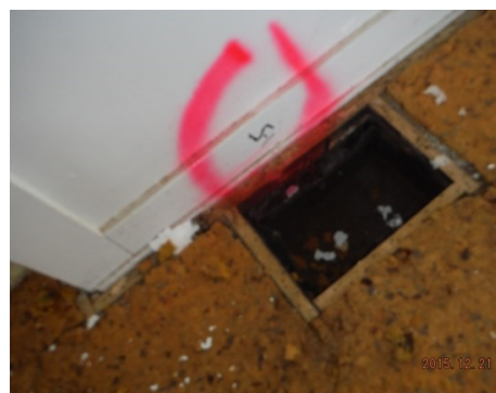
Sample 5-1 Duct Wrap
