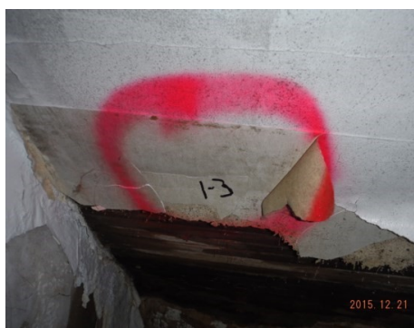
Sample 1-3 Plaster/Skim Coat
