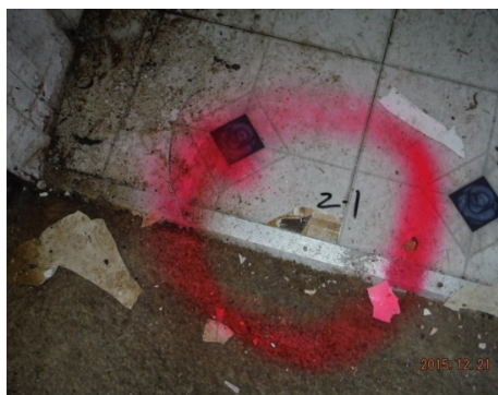
Sample 2-1 Floor Tile/Mastic
