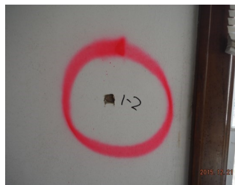
Sample 1-2 Plaster/Skim Coat
