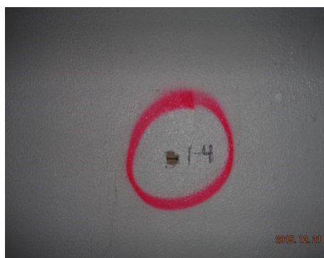
Sample 1-4 Plaster/Skim Coat
