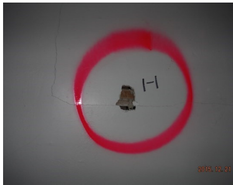
Sample 1-1 Plaster/Skim Coat
