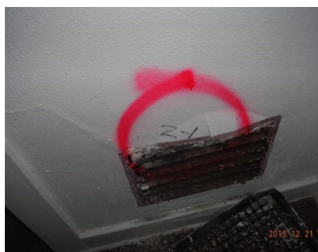
Sample 2-1 Duct Wrap
