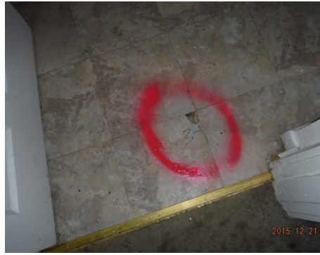
Sample 3-1 Floor Tile/Mastic
