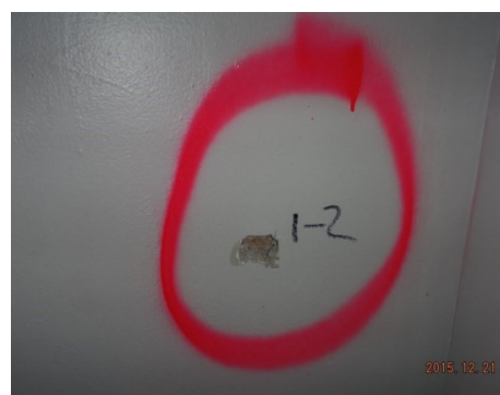
Sample 1-2 Plaster/Skim Coat
