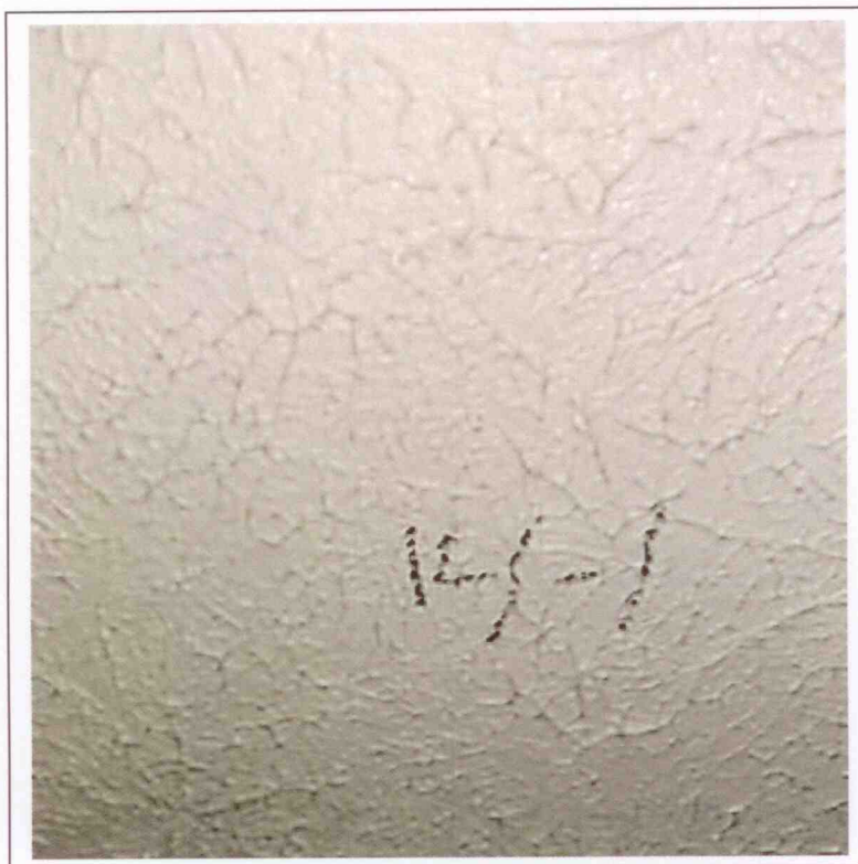
Textured ceiling, rough
