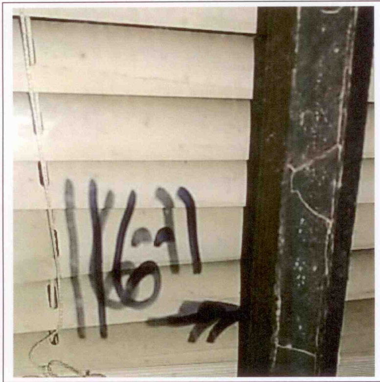
Exterior window glaze
