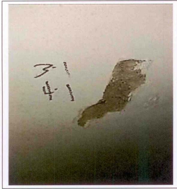
Hard wall and ceiling plaster
