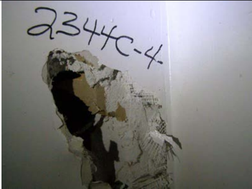
Photo 3: Drywall/J.C. (2344C-4) Living Room, Wall C. No Asbestos Detected.
