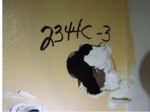
Photo 2: Drywall/J.C. (2344C-3) Bedroom 1, Wall B. No Asbestos Detected.
