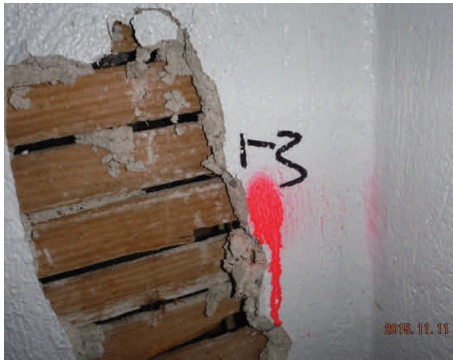
Plaster 1-3 Plaster/Skim Coat
