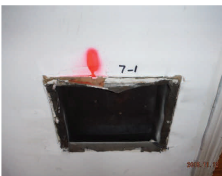
Sample 7-1 Duct Wrap
