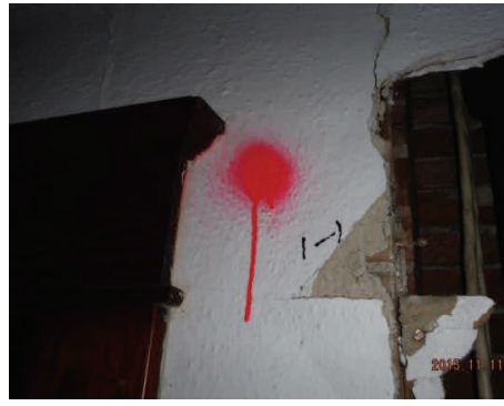
Sample 1-1 Plaster/Skim Coat
