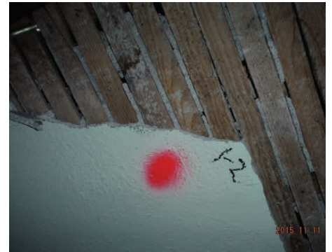
Sample 1-2 Plaster/Skim Coat
