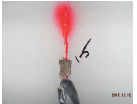
Sample 1-5 Plaster/Skim Coat
