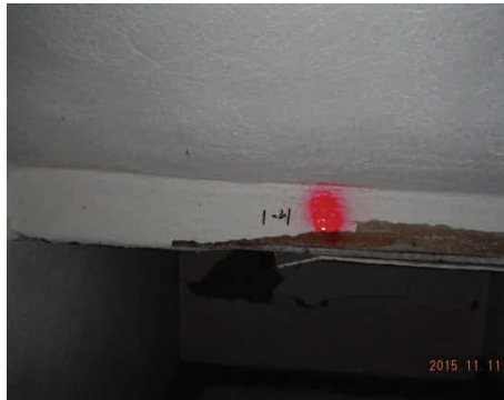
Sample 1-4 Plaster/Skim Coat
