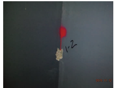
Sample 1-2 Plaster/Skim Coat
