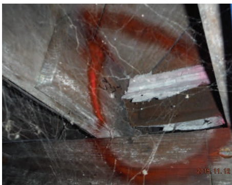
Sample 5-2 Duct Wrap
