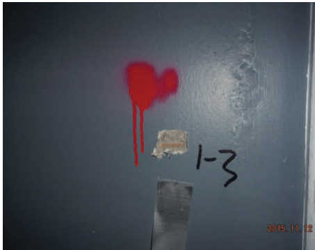
Plaster 1-3 Plaster/Skim Coat
