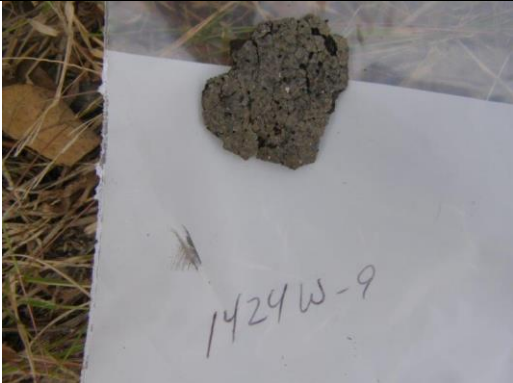
Photo 9: Roof Shingle (1424W-9) Exterior. No Asbestos Detected.
