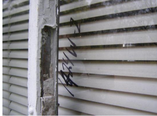
Photo 2: Window Glazing (1424W-2) Exterior, Wall A. 2% Chrysotile Asbestos Detected (PC=1.25%).
