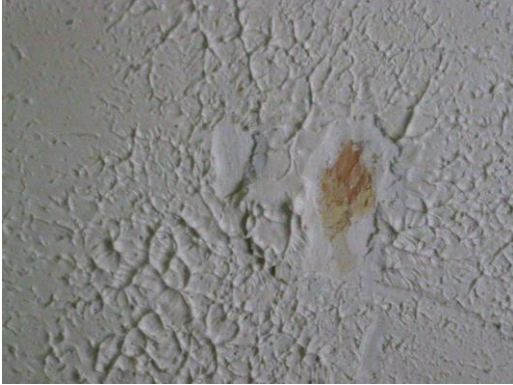
Photo 7: Textured Paint (1424W-7) Living Room, Ceiling. No Asbestos Detected.
