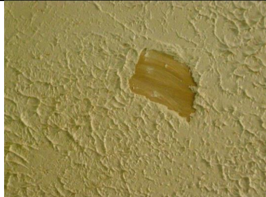
Photo 6: Textured Paint (1424W-6) Kitchen, Ceiling. No Asbestos Detected.
