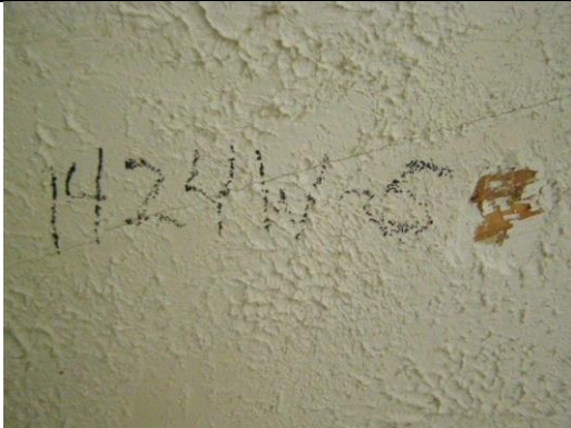
Photo 5: Textured Paint (1424W-5) Bath, Ceiling. No Asbestos Detected.
