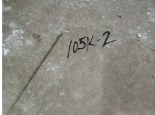
Photo 2: Tile (105K-2) Kitchen, Floor. 3% Chrysotile Asbestos Detected (PC=3.50%).
