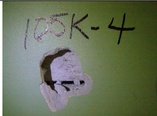
Photo 4: Plaster (105K-4) Kitchen, Wall A. Trace <1% Chrysotile Asbestos Detected (PC=<0.25%).
