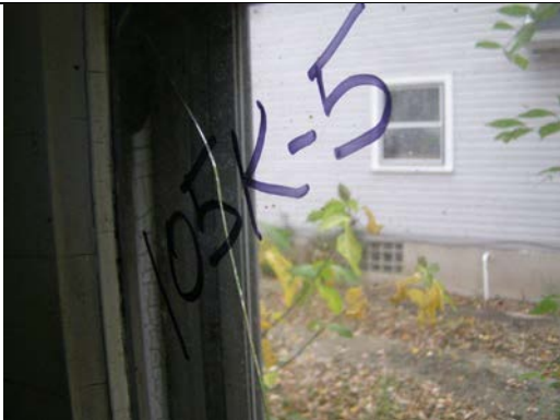
Photo 5: Window Glazing (105K-5) Kitchen, Wall B. No Asbestos Detected.
