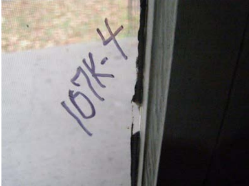
Photo 13: Window Glazing (107K-4) Living Room, Wall A. No Asbestos Detected.
