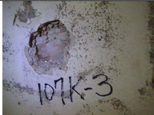
Photo 12: Plaster (107K-3) Living Room, Wall D. Trace <1% Chrysotile Asbestos Detected (PC=0.25%).
