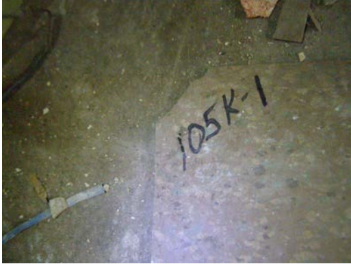
Photo 1: Tile(105K-1) Kitchen, Floor. 3% Chrysotile Asbestos Detected (PC=2.50%).
