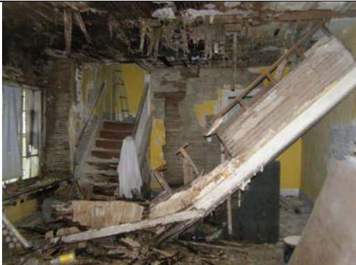
Photo 17: Interior view of 105 Knecht Dr.
