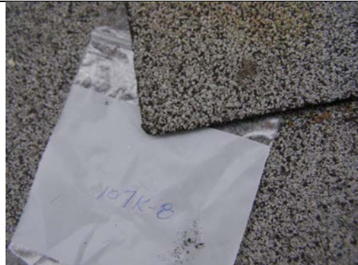
Photo 16: Roof Shingle (107K-8) Exterior. No Asbestos Detected.
