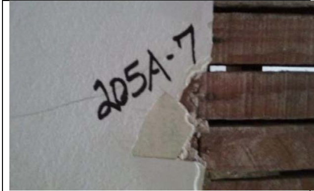
Photo 7: Plaster/Text. Pt. (205A-7) Hall, Wall B. Trace <1% Chrysotile Asbestos Detected (Plaster Texture PC=0.25%) (Plaster Base Coat PC=0.25%).
