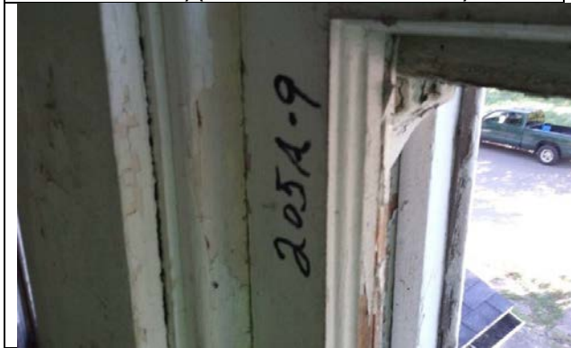
Photo 9: Window Glazing (205A-9) Bedroom 2, Wall A. Trace <1% Chrysotile Asbestos Detected (PC=0.25%).
