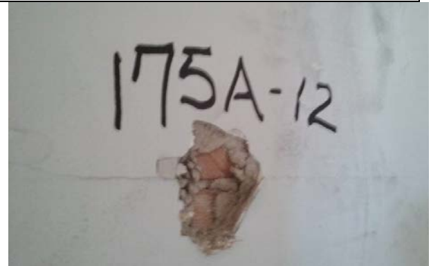
Photo 12: Plaster (175A-12) Bedroom 1, Closet. No Asbestos Detected.
