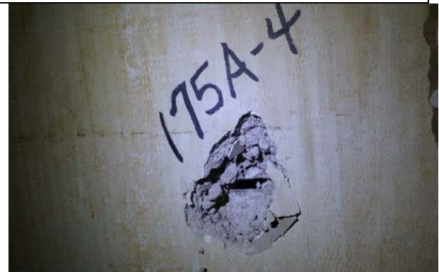
Photo 4: Plaster (175A-4) Family Room, Wall C. No Asbestos Detected.
