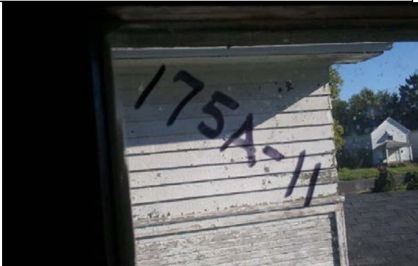
Photo 11: Window Glazing (175A-11) Bedroom 1, Wall D. No Asbestos Detected.
