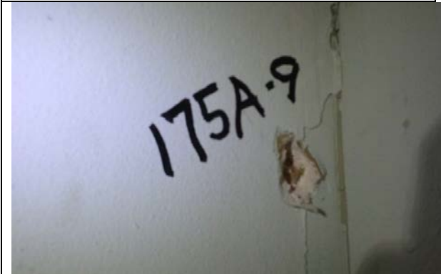
Photo 9: Drywall/J.C. (175A-9) Dining Room, Wall D. No Asbestos Detected.
