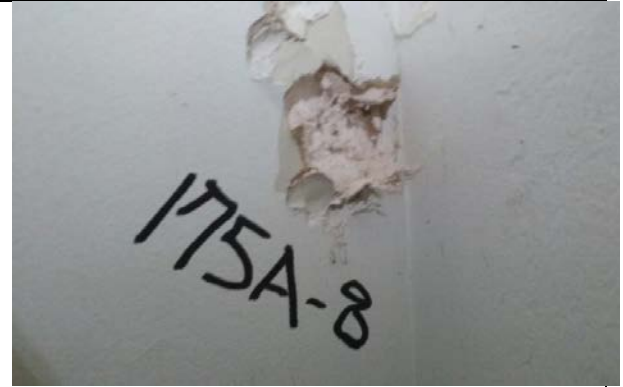
Photo 8: Drywall/J.C. (175A-8) Living Room, Wall A. No Asbestos Detected.
