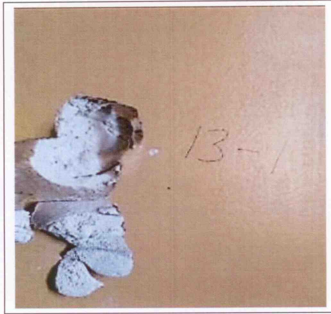
HA #13 – Drywall, new
