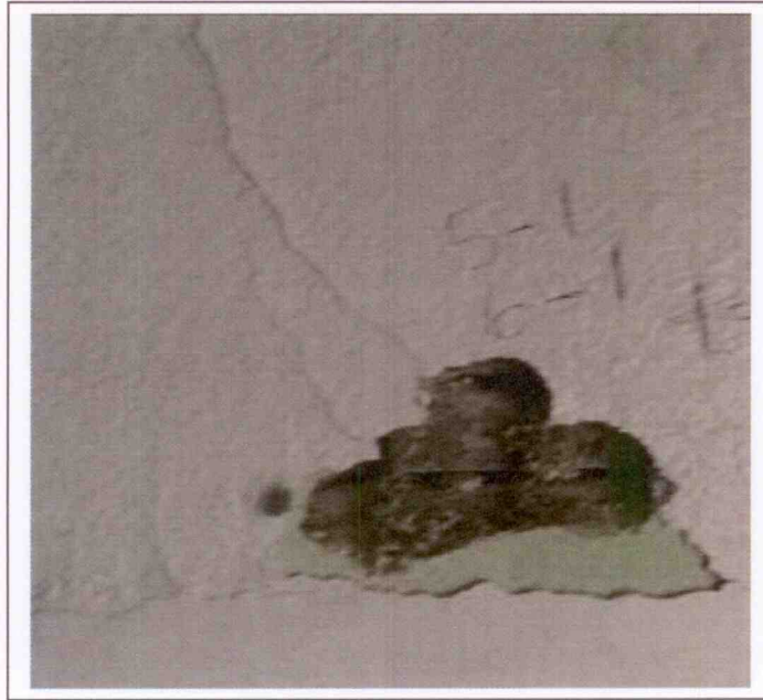
HA #5 & #6 – Hard wall and ceiling plaster
