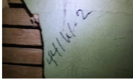
Photo 2: Plaster (441W-2) Basement Steps, Wall C. Trace <1% Chrysotile Asbestos Detected (PC=0.25%).
