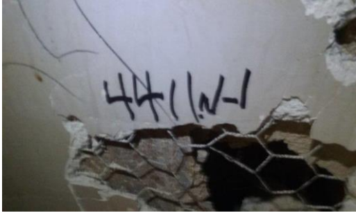
Photo 1: Plaster (441W-1) Kitchen, Wall C. Trace <1% Chrysotile Asbestos Detected (PC=0.50%).
