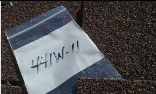
Photo 11: Roof Shingle (441W-11) Exterior. No Asbestos Detected.
