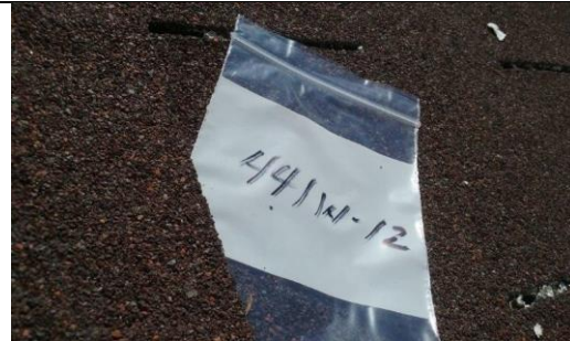
Photo 12: Roof Shingle (441W-12) Exterior. No Asbestos Detected.
