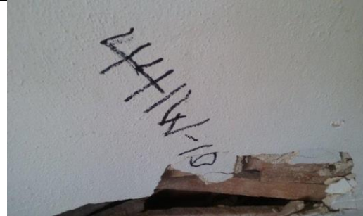
Photo 10: Plaster (441W-10) Bedroom 2, Wall D. Trace <1% Chrysotile Asbestos Detected (PC=0.50%).
