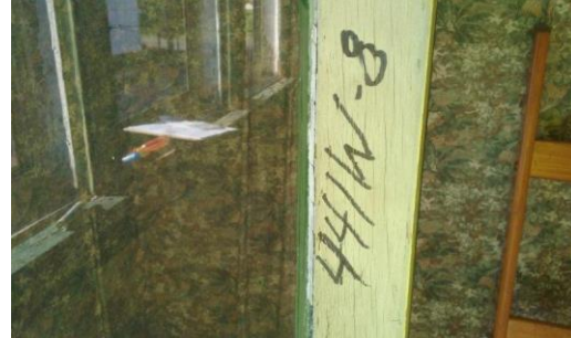
Photo 8: Window Glazing (441W-8) Bedroom 1, Wall C. Trace <1% Chrysotile Asbestos Detected (PC=0.25%).
