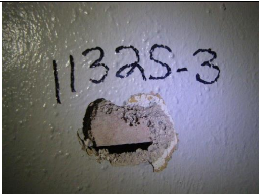
Photo 3: Plaster (1132S-3) Living Room, Wall D. No Asbestos Detected.
