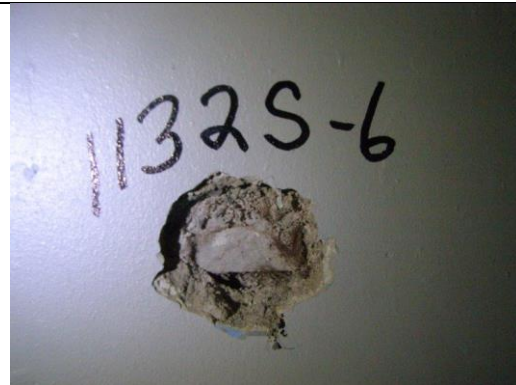
Photo 6: Plaster (1132S-6) Bedroom 3, Wall B. No Asbestos Detected.
