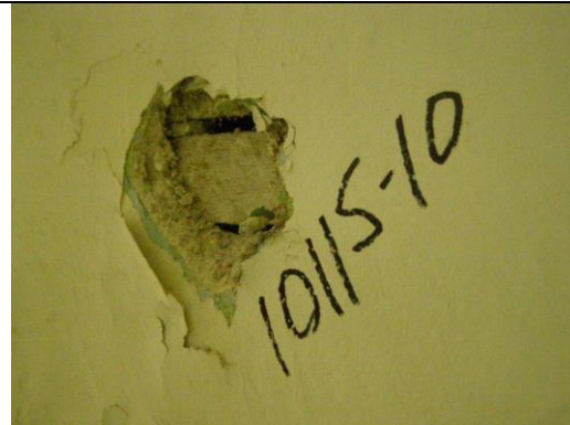
Photo 10: Plaster (1011S-10) Bedroom 2, Wall B. No Asbestos Detected.
