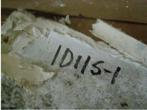
Photo 1: Drywall/J.C. (1011S-1) Family Room, Ceiling. No Asbestos Detected.
