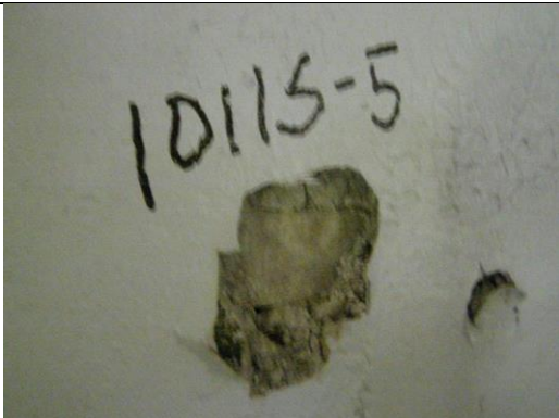
Photo 5: Plaster (1011S-5) Living Room, Wall C. No Asbestos Detected.
