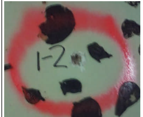
Sample 1-2 Drywall/Joint Compound
