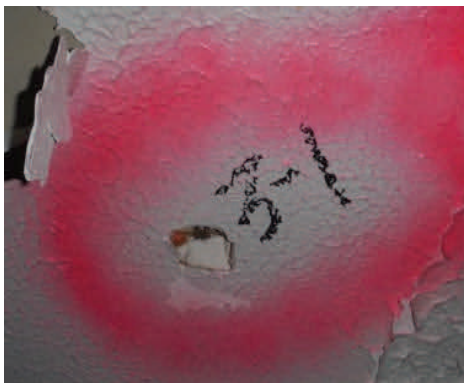
Sample 3-1 Drywall w/ Skim Coat
