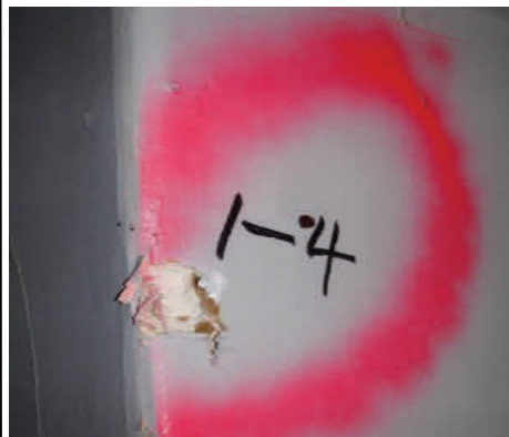
Sample 1-4 Drywall/Joint Compound
