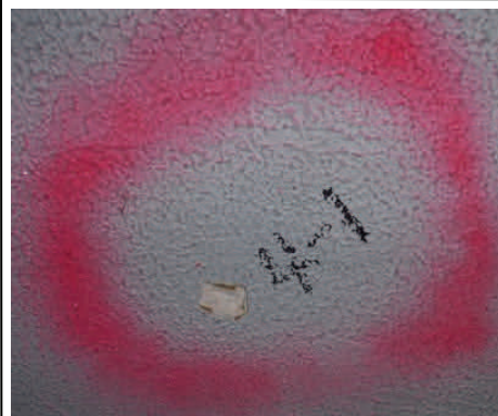
Sample 4-1 Drywall w/ Skim Coat
