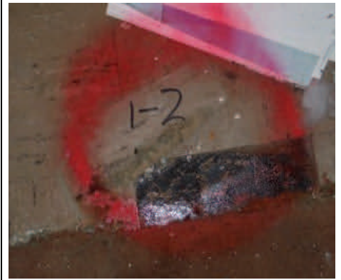
Sample 1-2 Floor Tile/Mastic
