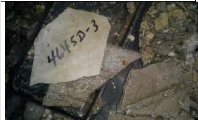
Photo 3: Plaster (4645D-3) Living Room, Ceiling. Trace <1% Chrysotile Asbestos Detected (PC=0.25%).
