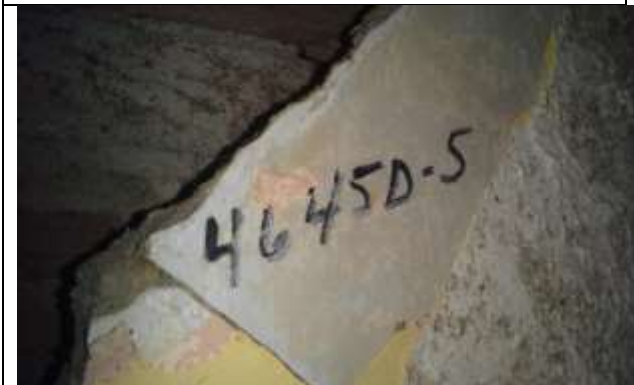
Photo 5: Plaster (4645D-5) Kitchen, Wall A. Trace <1% Chrysotile Asbestos Detected (PC=<0.25%).
