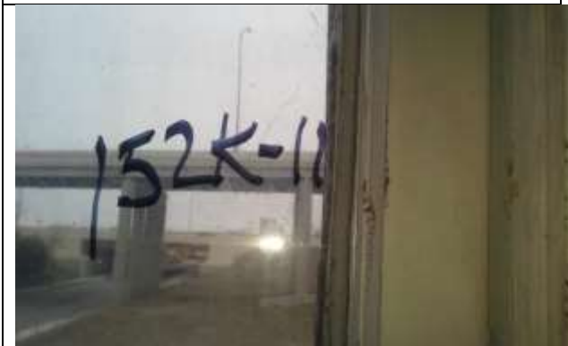
Photo 11: Window Glazing (152K-11) Bedroom 1, Wall A. No Asbestos Detected.
