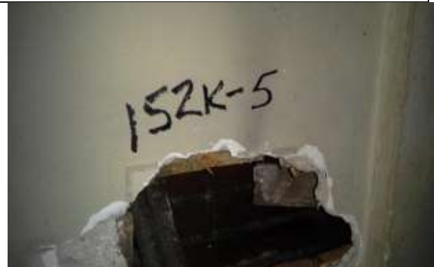
Photo 5: Plaster (152K-5) Dining Room, Wall B. No Asbestos Detected
