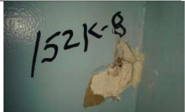
Photo 8: Drywall/J.C. (152K-8) Bath 1, Wall D. No Asbestos Detected.
