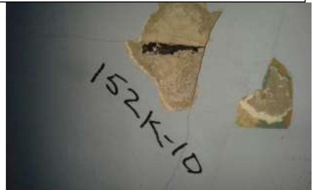
Photo 10: Plaster (152K-10) Bedroom 1, Wall C. No Asbestos Detected.
