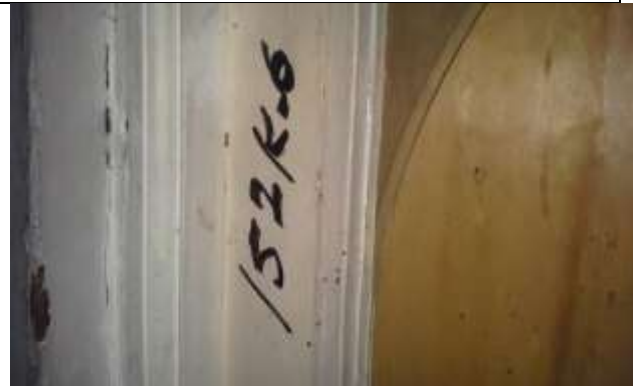
Photo 6: Window Glazing (152K-6) Dining Room, Wall D. No Asbestos Detected
