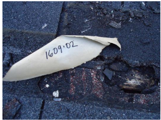
Photo 2: Roofing, (1609-2) Roof. No Asbestos Detected.
