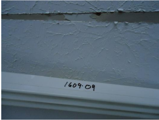
Photo 9: J.C. (1609-9) Room 1 West Wall. No Asbestos Detected.
