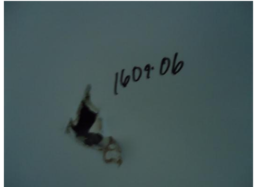
Photo 6: Drywall (1609-6) Room 3 East Wall. No Asbestos Detected.
