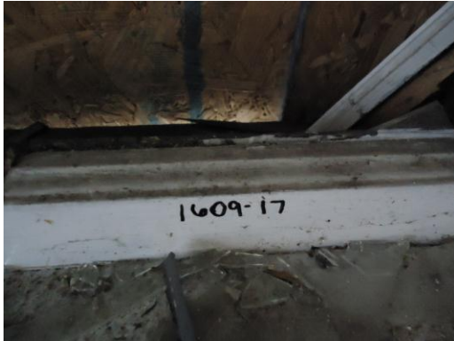
Photo 17: Window Caulk (1609-17) Living Room East Wall. No Asbestos Detected
