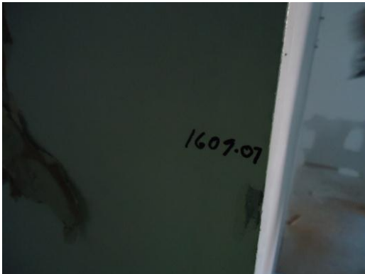
Photo 7: J.C. (1609-7) Bath East Wall. No Asbestos Detected.
