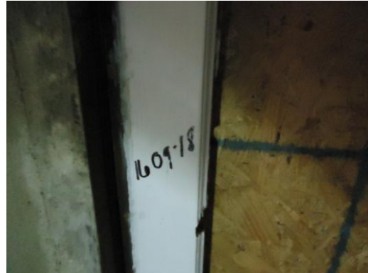
Photo 18: Window Caulk (1609-18) Room 5 South Wall. No Asbestos Detected
