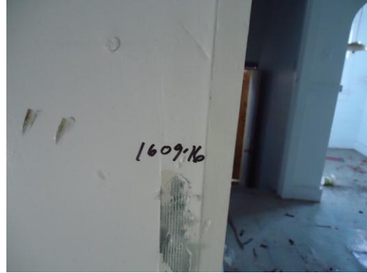
Photo 16: J.C. (1609-16) Kitchen West Wall. No Asbestos Detected.
