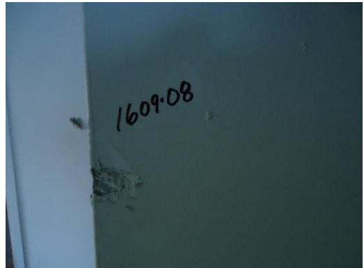
Photo 8: J.C. (1609-8) Hallway West Wall. No Asbestos Detected.
