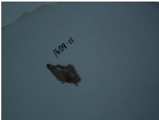
Photo 11: Ceiling Plaster (1609-11) Dining Room. No Asbestos Detected.
