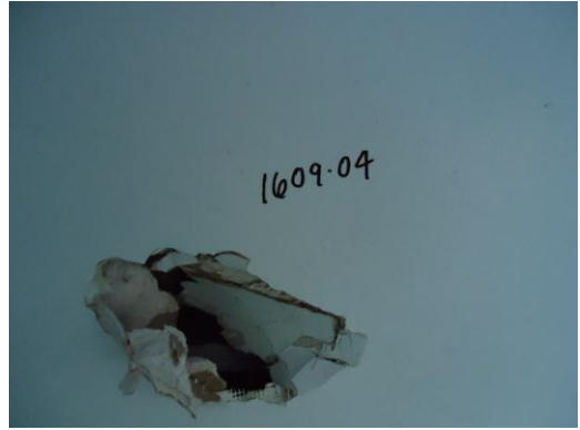
Photo 4 Drywall (1609-4) Room 1 West Wall. No Asbestos Detected.
