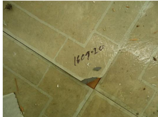
Photo 20: Floor Tile (1609-20) Kitchen. No Asbestos Detected
