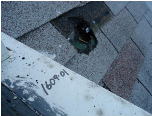
Photo 1: Roofing, (1609-1) Roof. No Asbestos Detected.
