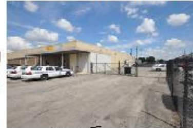
East POD – North - 417 E. Helena Street
