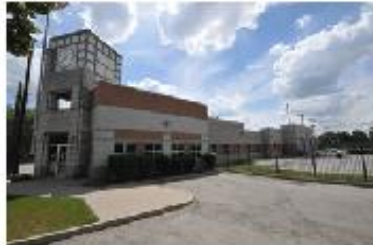
Central POD - 248 Salem Avenue
