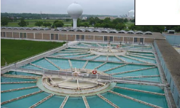
Miami Water Treatment Plant
