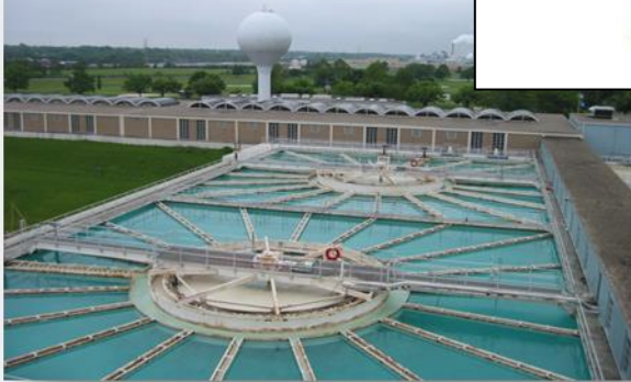
Miami Water Treatment Plant
