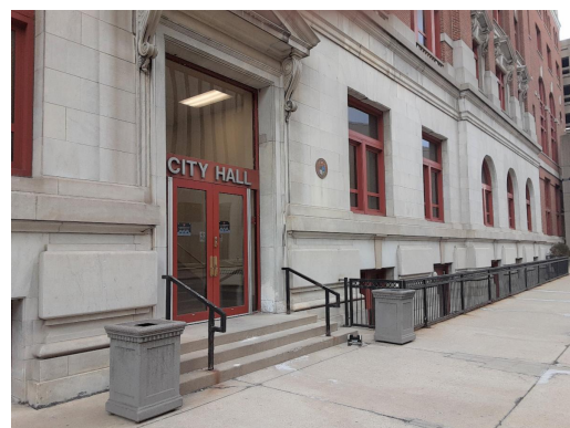
City Hall: Current Ludlow Street entrance
