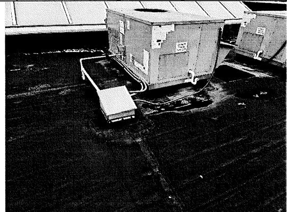
40 – Typical rooftop unit and equipment enclosure
