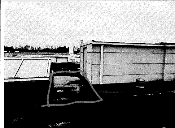
35 – EPDM roof system is soft [insulation is breaking down] between the end of the roof monitor and the skylight at the roof access door
