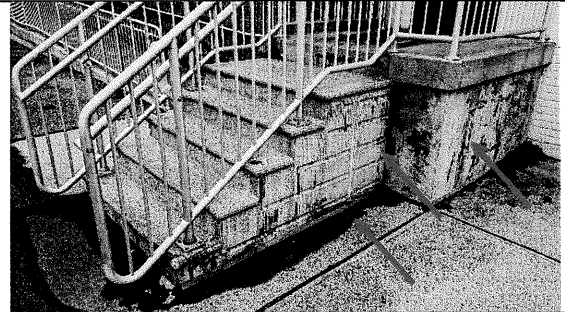
28 – Southeast Stair / Landing -
