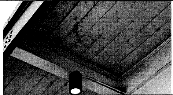
10 – Underside of roof canopy / overhang -
