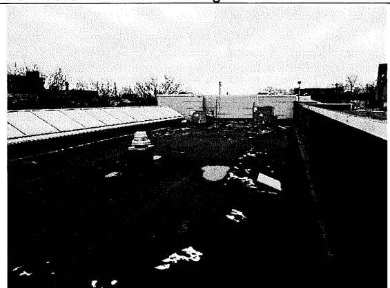
30 – Main Building Roof looking East, south warehouse roof is to the right of the photo.
