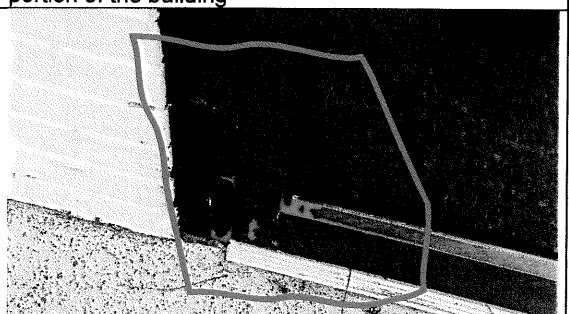
08 – aluminum storefront system – painted finishes are failing exposing the original colored anodized finish
