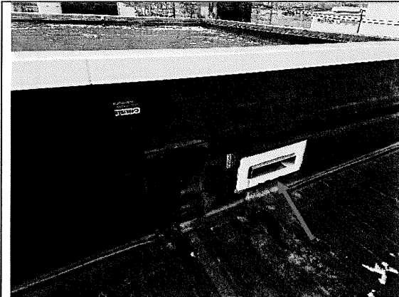
43 – Drainage scupper thru the intersecting parapet wall between the East Warehouse and the original building roof for drainage of the east warehouse. Note rusting on the metal
