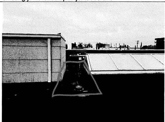
34 – EPDM roof system is soft [insulation is breaking down] between the end of the roof monitor and the skylight.
