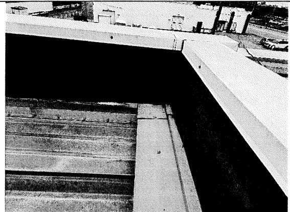
46 – EPDM wase flashing over CMU parapet walls, capped with metal coping at south warehouse roof.
