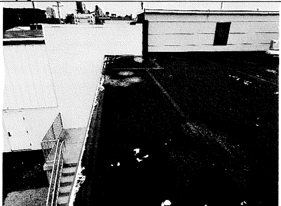
36 – Roof edge at the south side of the original building looking west
