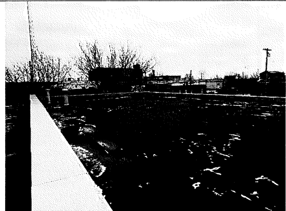
42 – East warehouse roof, note sloped to the west toward the original portion of the building
