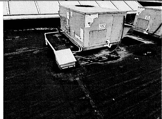
40 – Typical rooftop unit and equipment enclosure
