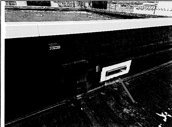
43 – Drainage scupper thru the intersecting parapet wall between the East Warehouse and the original building roof for drainage of the east warehouse. Note rusting on the metal
