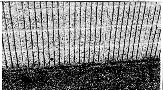
06 – Typical ribbed CMU at planters at base of original portion of the building
