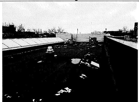
30 – Main Building Roof looking East, south warehouse roof is to the right of the photo.
