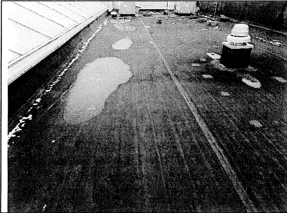
31 – Main Building Roof looking East
