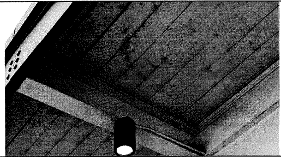
10 – Underside of roof canopy / overhang -
