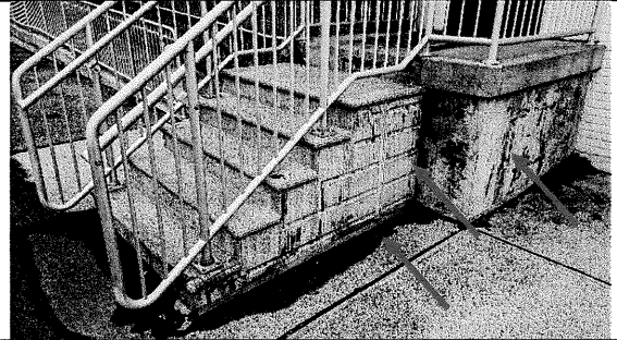
28 – Southeast Stair / Landing -
