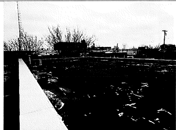
42 – East warehouse roof, note sloped to the west toward the original portion of the building
